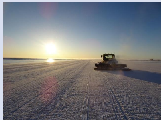
Final runway surface preparations at Wilkins Aerodrome. Photo courtesy M Ryan.
