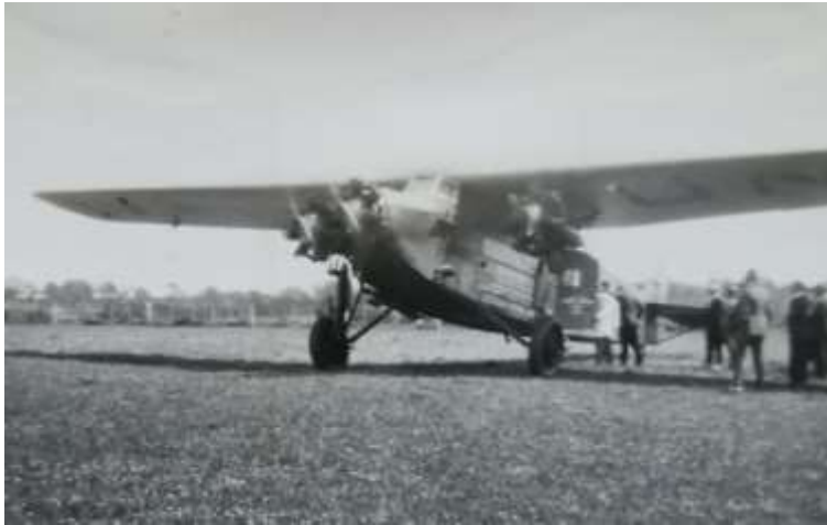
The Southern Sun at Western Junction
