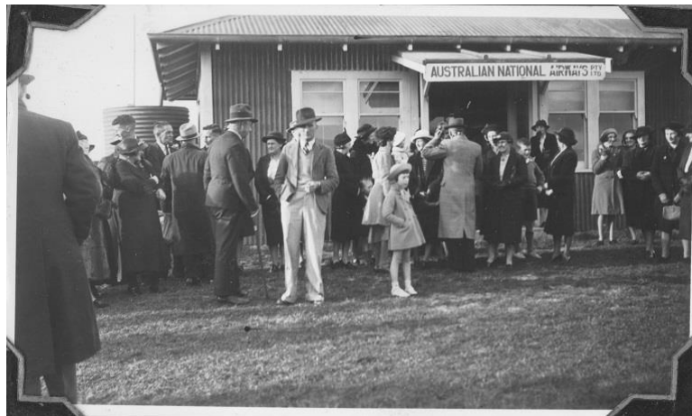
ANA Building at St Pats River Aerodrome (Photo compliments of the Brammall family.)
