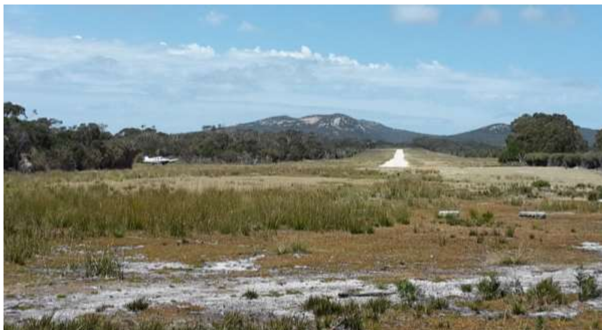
Killiecrankie airstrip Flinders Island, the proposed destination of VH-WMD. The airstrip is 1300 metres in length, sandy based and is aligned 09/27. It has no navigational aids.
