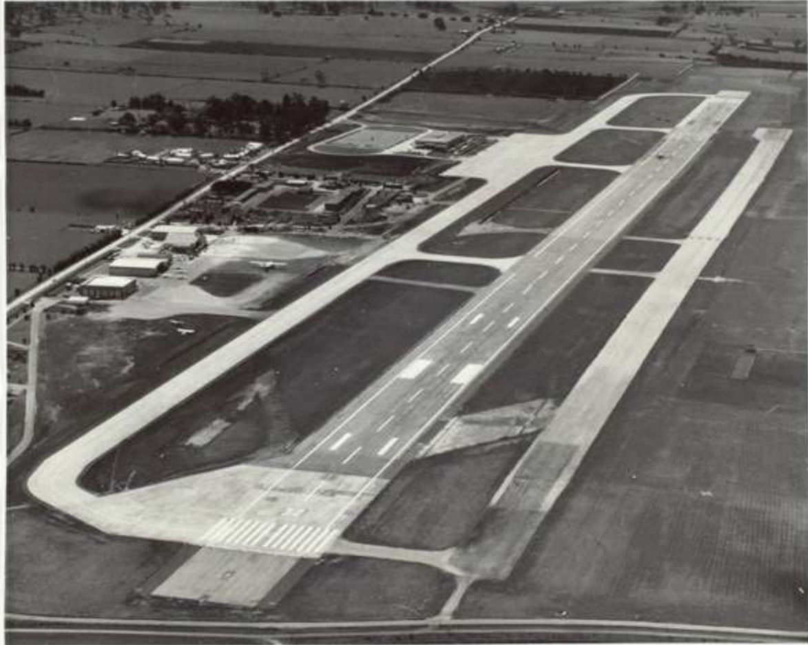
Western Junction about 1968, with the new terminal at the northern end (top)
